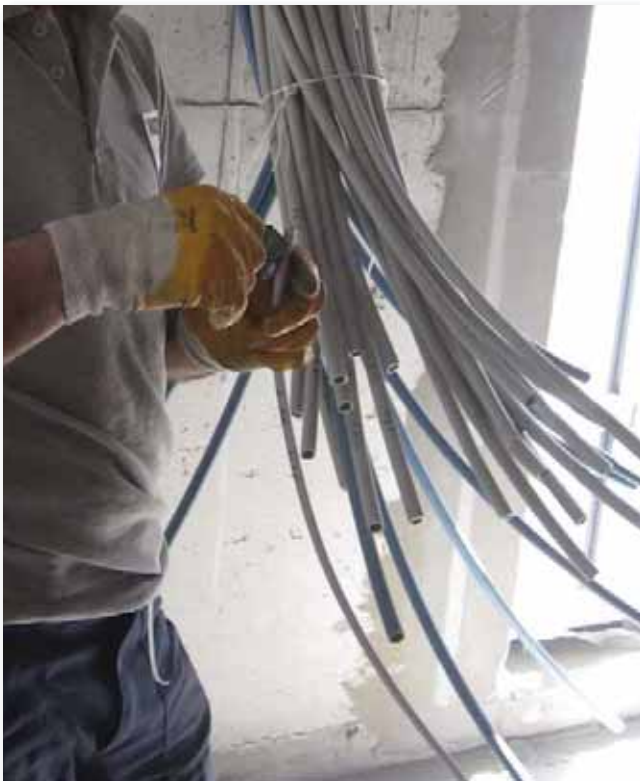
An operator stripping cables during installation.
