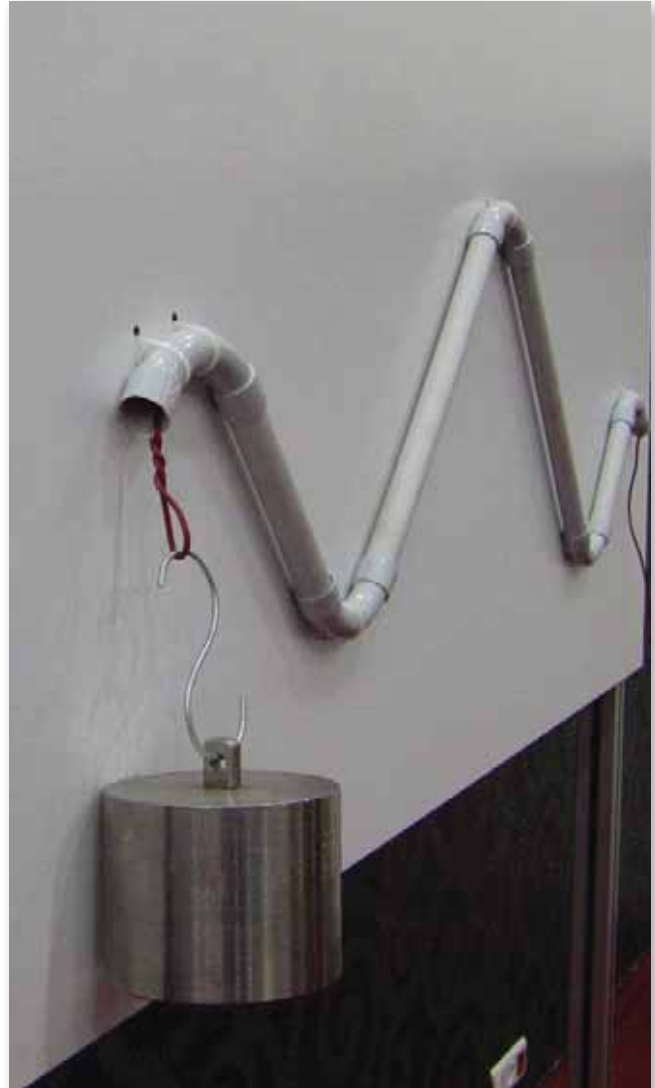
Slippery cables can move through ducts even with small amount of force.
